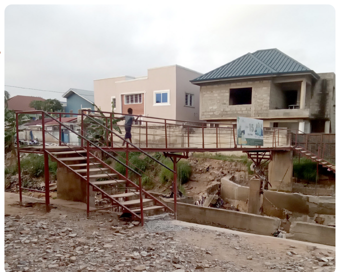
Bridge across drainage canal, Dome, Accra
