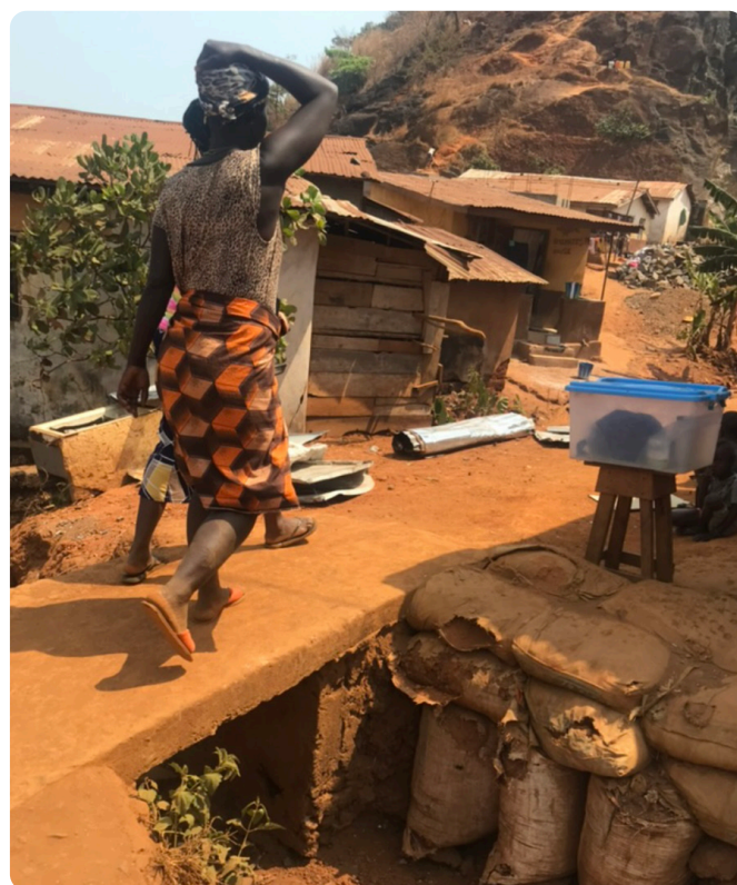
Bridge across drainage canal, Moyiba, Freetown
