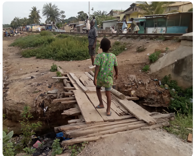
Bridge across gutter, Dome, Accra
